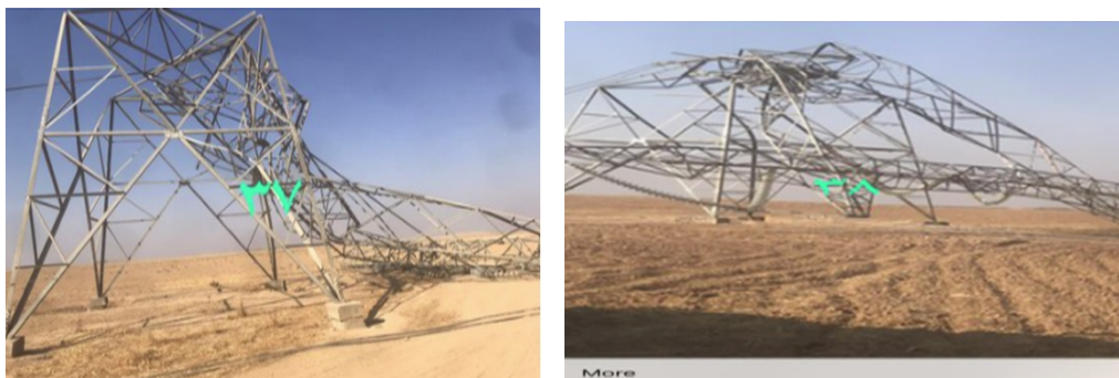
High-voltage pylons of the main power line hit by the detonation of IEDs (Iraqi News Agency, November 24, 2020)
