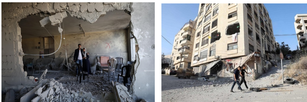
The apartment demolished by Israeli security forces (Right: @J7Rahaf Twitter account. Left: Wafa, June 22, 2023).
