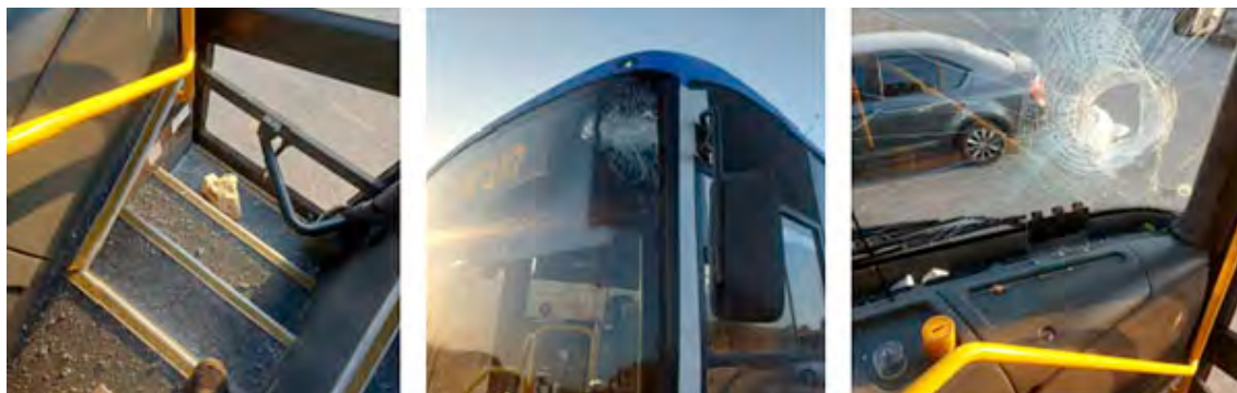
Right: The damage to the bus attacked near Nebi Elias (east of Qalqilya). Left: A rock thrown at the bus.
