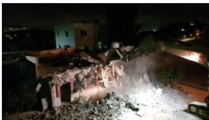
Demolition of the terrorist's house (IDF spokesman's X account, November 15, 2023)
