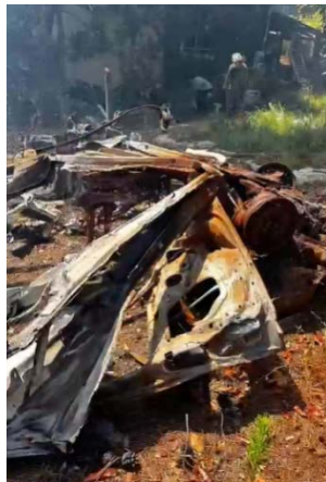
Damage from a direct hit (Upper Galilee Regional Council spokesman's unit, July 25, 2024)
