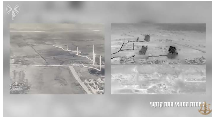
Destruction of the tunnel in the central Gaza Strip (IDF spokesperson, August 28, 2024)
